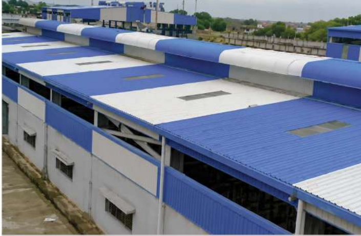
L&T, CENTRAL RAILWAY, JHANSI, AREA: 10,530 SQM
