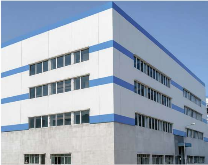
BHAVNAGAR, GUJARAT, PLANT AREA: 19,000 SQM
