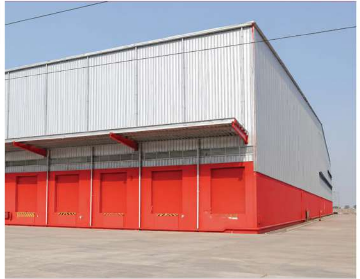
BHIWANDI, MAHARASHTRA, PLANT AREA: 28,000 SQM
