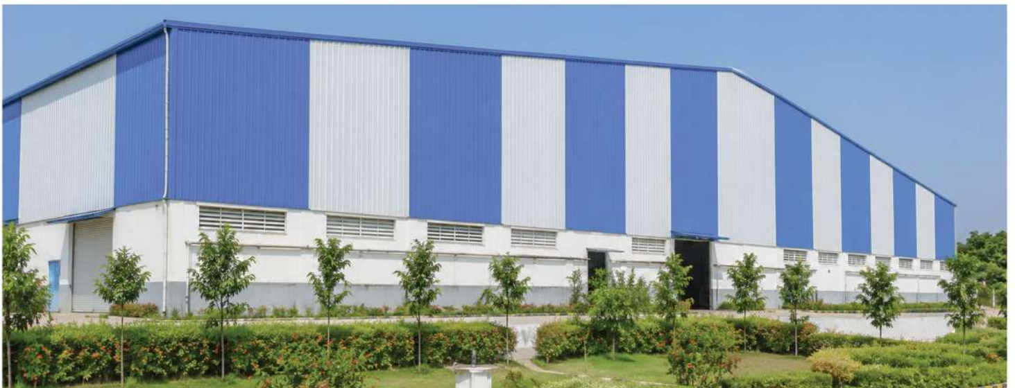
TURNKEY PROJECT, PANIPAT, AREA: 18,116 SQM
