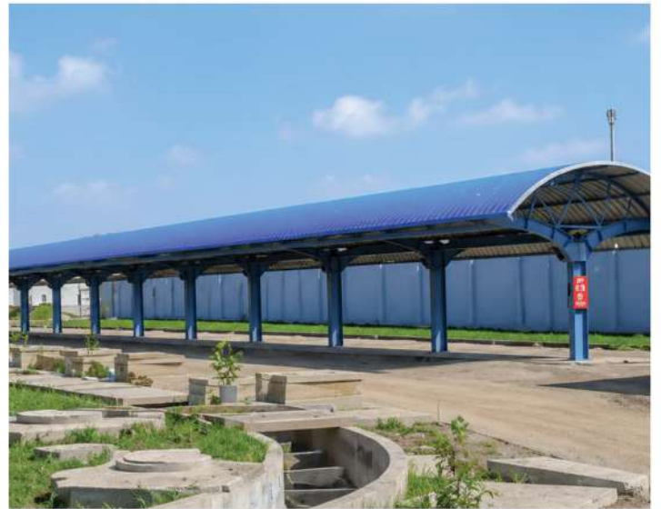
DMRC CAR SHED AT FARIDABAD
