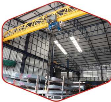
Heavy Fabrication Bays with crane support
