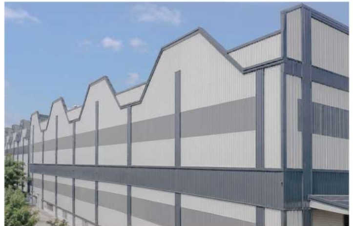
AURANGABAD, MAHARASHTRA BUILDING
